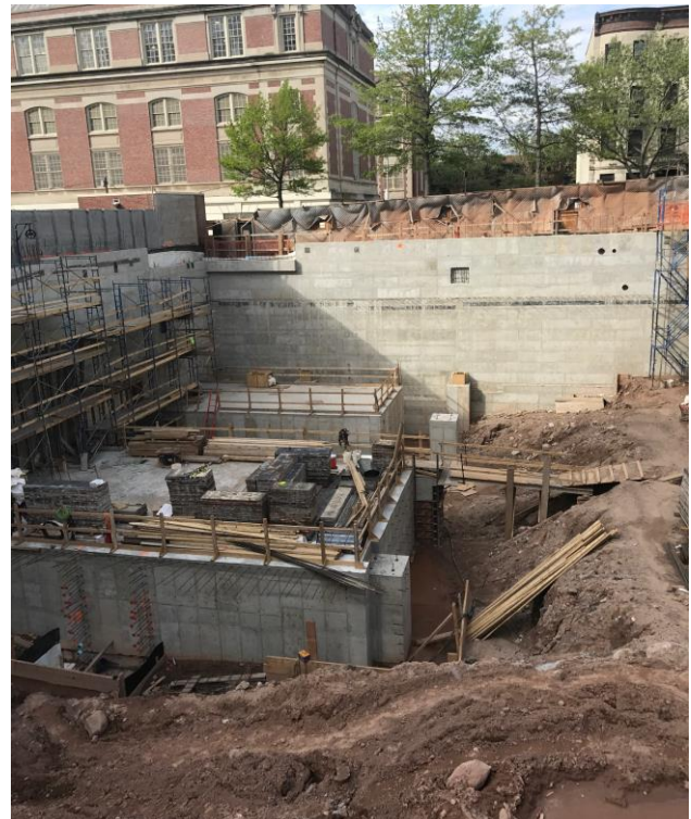
Cast-in-place concrete fire and storm tanks and north west foundation walls
