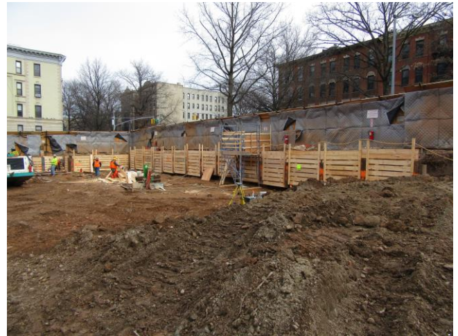
An inside view: Support of Excavation along Eighth Avenue.
