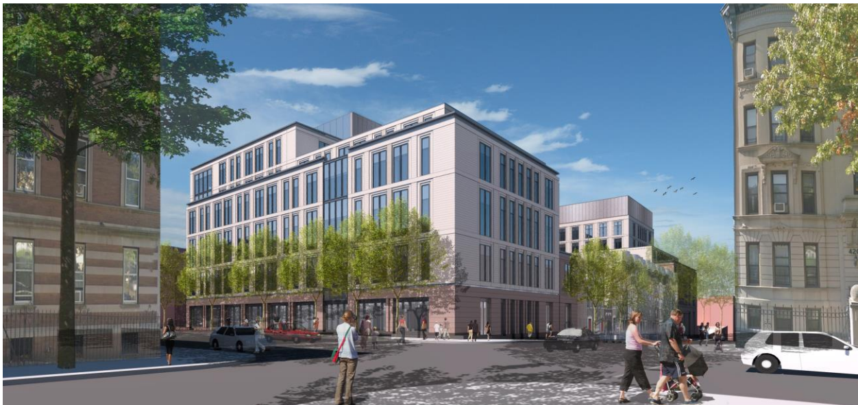
The Center for Community Health, viewed from the corner of Eighth Avenue and Fifth Street (Perkins Eastman)
