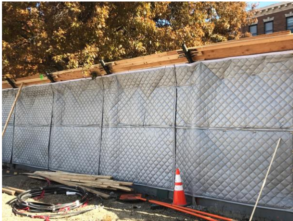
Construction fence with acoustic blankets lining the inside to mitigate sound.
