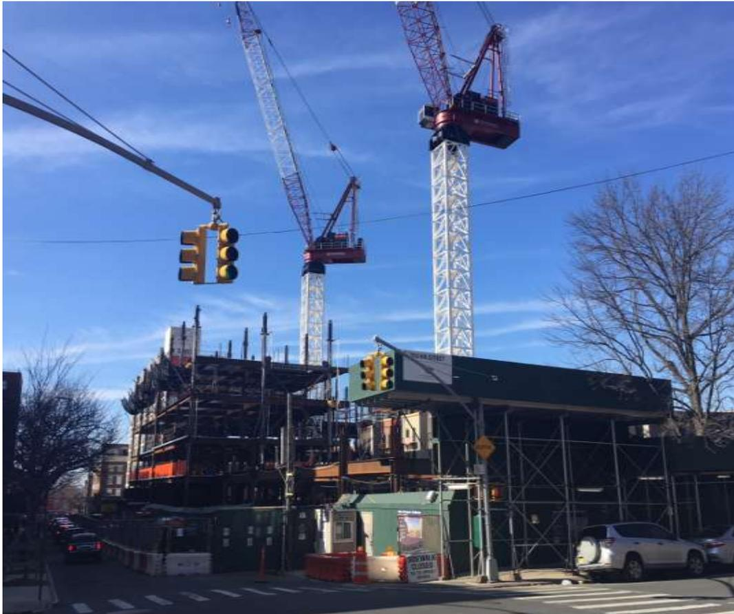
Both of the tower cranes are operational and steel installation is ongoing. As was the case with the first tower crane, the arrival of the second crane was delayed due to revisions of the Department of Buildings (DOB) tower crane protocols. The logistics on Sixth Street will continue to be implemented and will continue to be extended as needed to accommodate this phase of the project.
