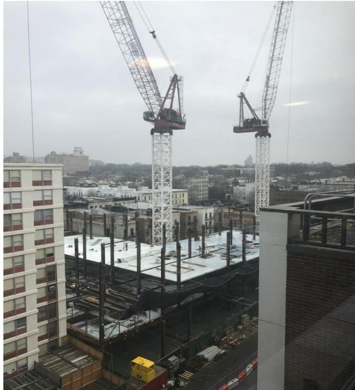
Both of the tower cranes are operational and steel installation is ongoing. As was the case with the first tower crane, the arrival of the second crane was delayed due to revisions of the Department of Buildings (DOB) tower crane protocols. The logistics on Sixth Street will continue to be implemented and will continue to be extended as needed to accommodate this phase of the project.
