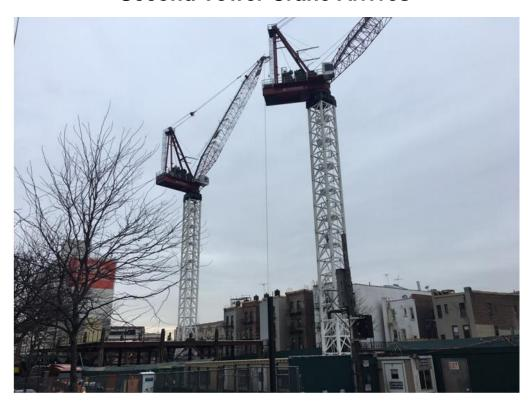
The second of the two tower cranes is being assembled and steel installation is set to continue. As was the case with the first tower crane, the arrival of the second crane was delayed due to revisions of the Department of Buildings (DOB) tower crane protocols. The logistics on Sixth Street will continue to be implemented and will likely be extended as needed to accommodate this phase of the project.
